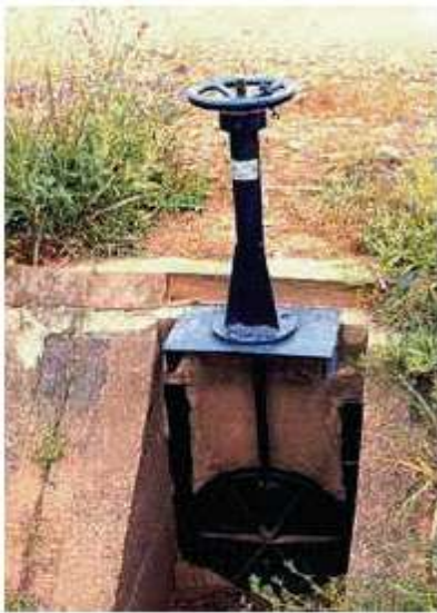
Left: a gate for a farm turnout. Right: a Neyropic gate.
