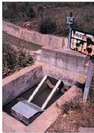
Left: a gate for a farm turnout. Right: a Neyropic gate.
